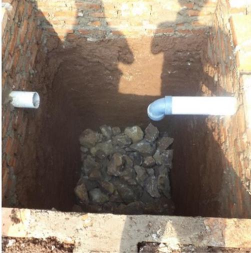
(a) Pipa *Outlet* Sumur Resapan
