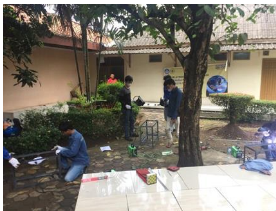
Figure 5. Welding project work process.
