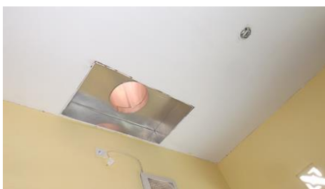
Figure 5. Ceiling and lighting
