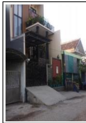
Figure 11. Raising the Floor of The House
