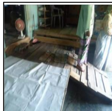
Figure 12. Raised the Floor of the House with Assembled Wood
