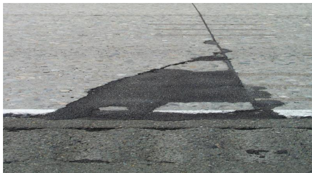
Figure 5. Patch Damage
