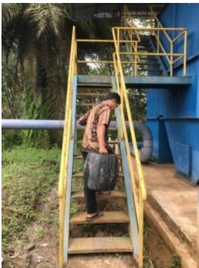
Figure 3. Carrying PAC liquid to top of WTP
