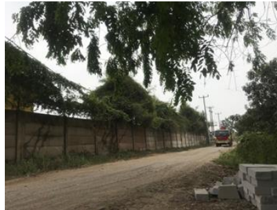
Figure 1. Soil condition at Kubang Laban Road, Serang.
