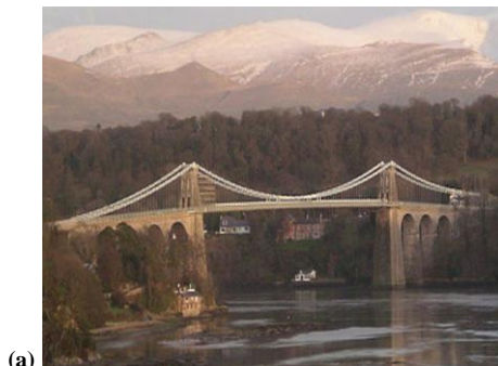
Figure 2 (a) Menai Straits Bridge, England
