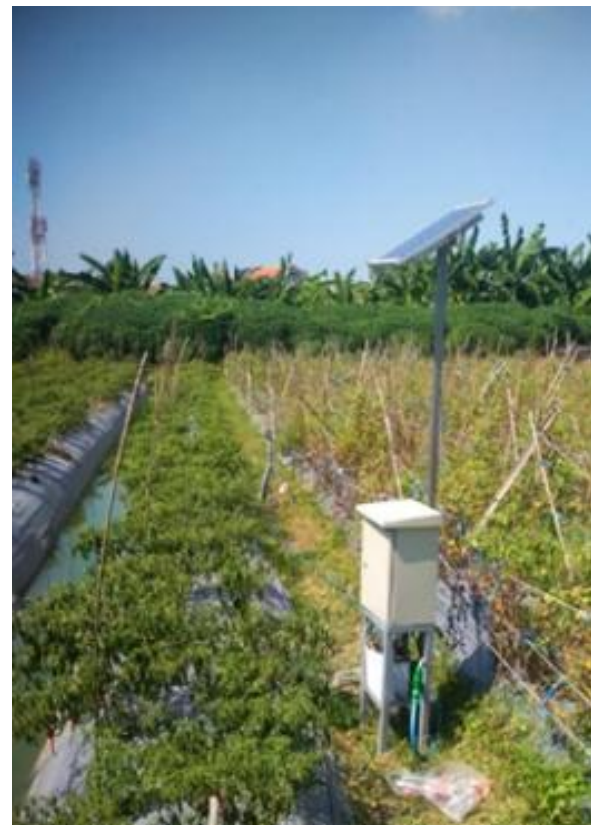
Figure 2. Installation of Smart Farming Devices works in off-grid area.
