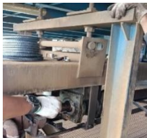
Figure 13. Replacement Gland Packing
