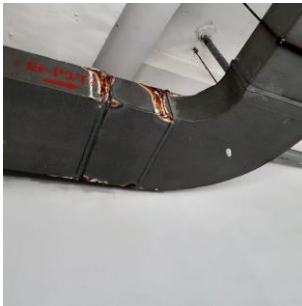
Figure 2. Ducting Corrosion
