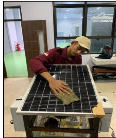
Figure 7. Electrical system maintenance
