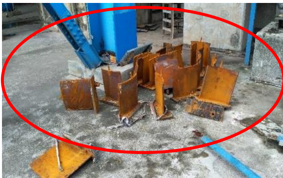
Figure 6. Damage to Static Blade
