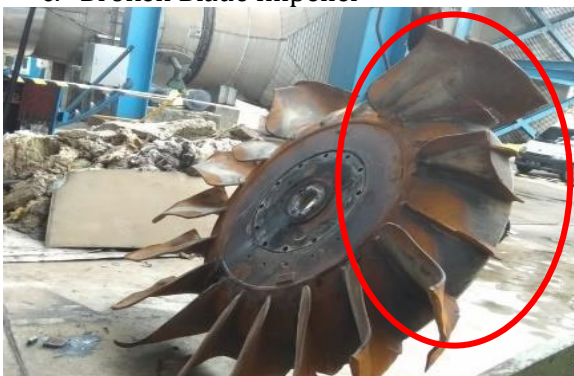
Figure 7. Damage to the Blade Impeller
