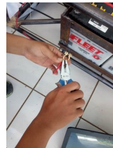
Figure 24. Linking MCB with Watt Meter Input
